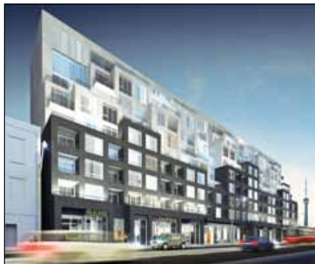
Changes on our doorstep: B-Street condos is a new development slated for the east side of Bathurst Street south of Bloor
